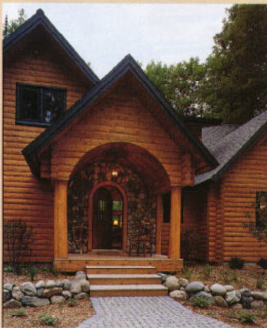
Half-log siding on the home's exterior is completed with full-log corners.
